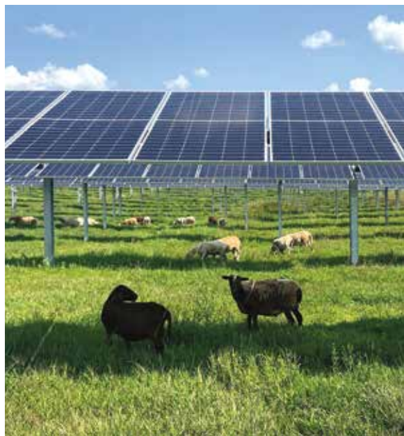
Blue Prairie Solar Project in Wisconsin produces approximately 5,000 MWh/year with surrounding vegetation beneficial to the landowner’s sheep and bees.
